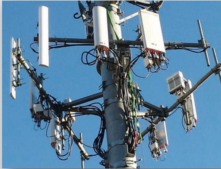
Panel Antennas with RRU's
