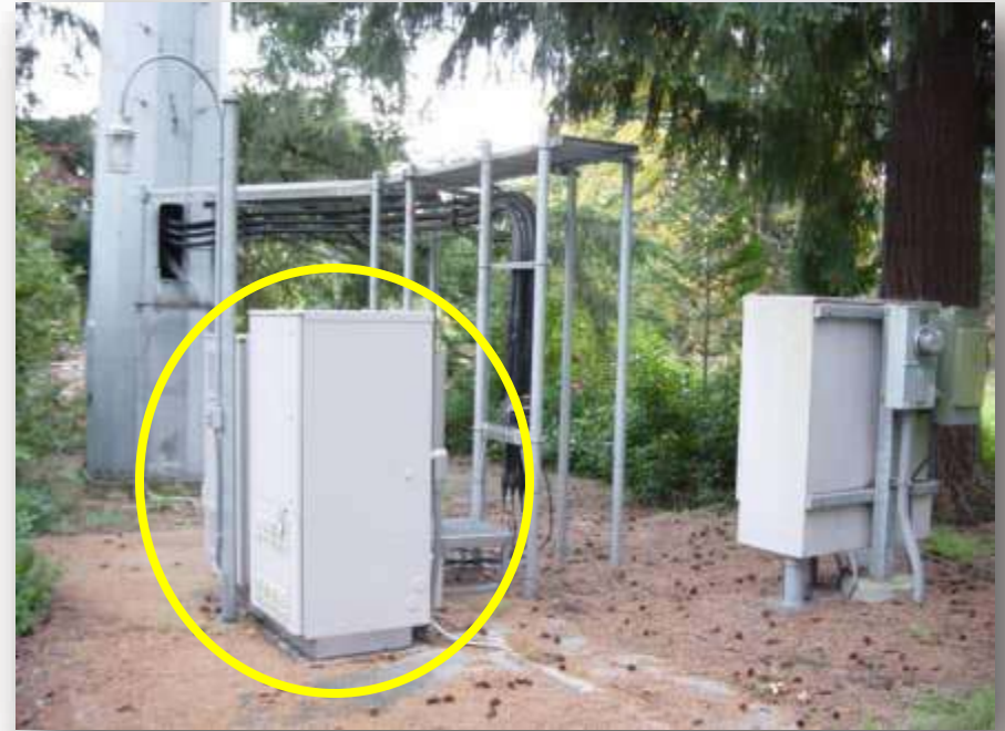
Typical High Frequency (1900-2400 MHz) Ground Equipment
