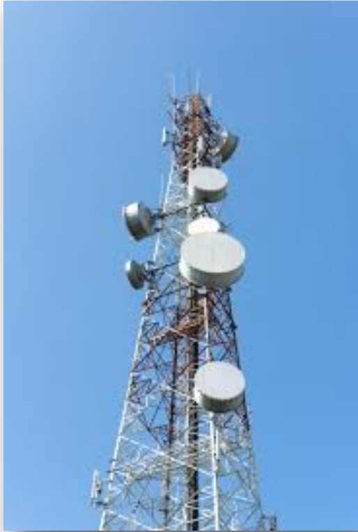
Microwave commonly used for backhaul
