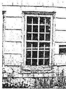
12/12 double-hung sash with 4-pane storm sash
